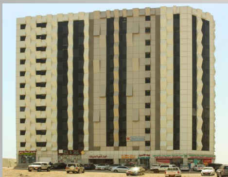
RES & COM BUILDING MABELA
