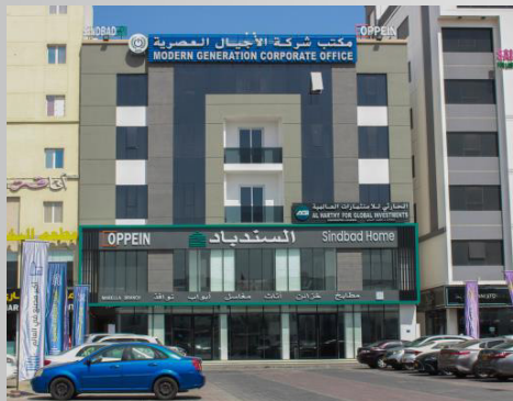
RES & COM BUILDING MABELA
